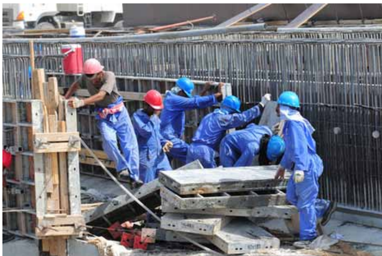
Figure 4. Problems is Maintaining Social Distance at Construction Site
