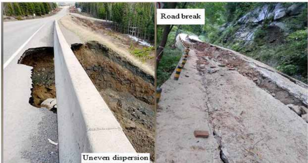
Figure 2. Local settlement of cement factor
