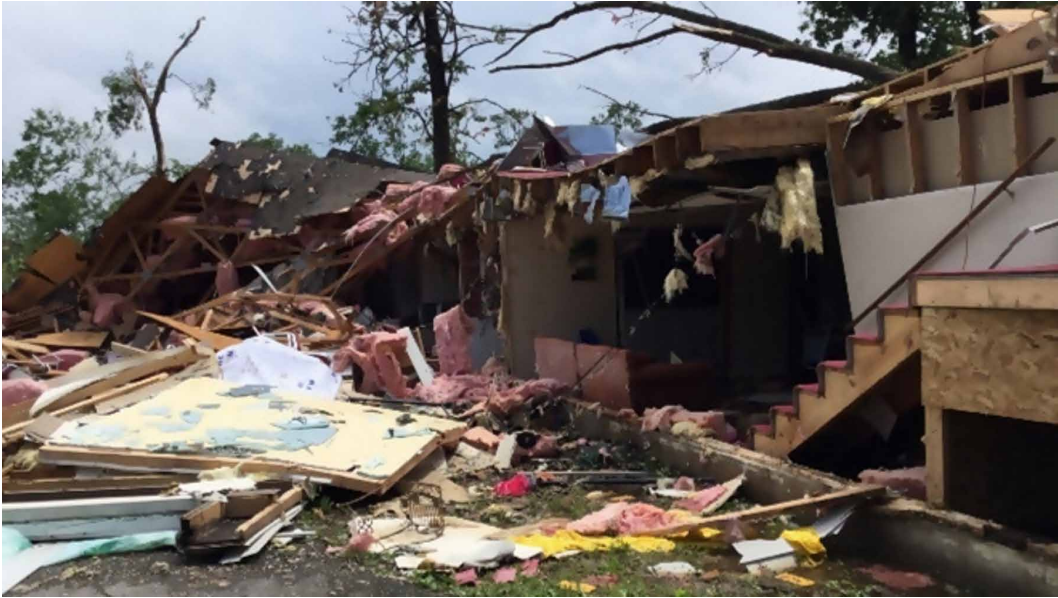
Figure 4. Walls collapsed by 150 mph winds around 11:33 PM in Jefferson, Missouri (NWS, 2019)
